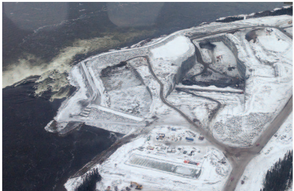
Figure 4 Site of Muskrat Falls Powerhouse and Spillway (2013)
